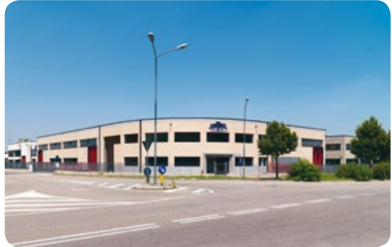
Nuovi reparti (lato sud) - New plant (from south)
